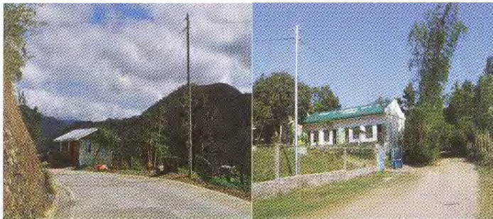
A house at the top of the mountain in Sitio Nompolia, Hungduan, Ifugao and a school in a far-flung area in Sitio Malipayon, Sagay City, Negros Occidental are among the beneficiaries of electricity from the government's Sitio Electrification Program (SEP).
